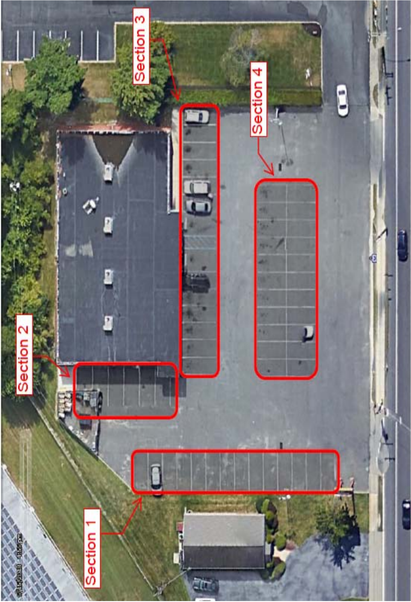
162 NJSH Route 49 Pennsville Township, Salem County, New Jersey
